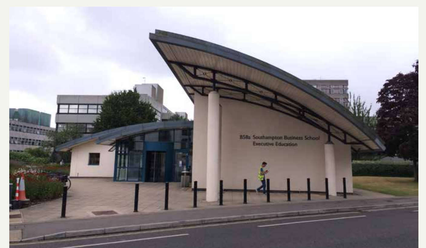
Existing building 58A
